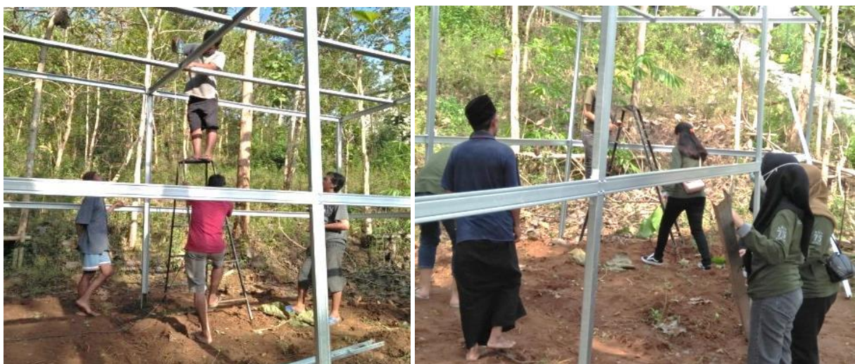
Picture 10. Light Steel Paranet Installation
