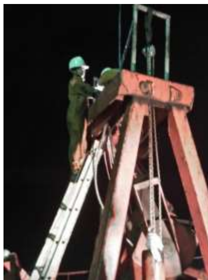
Figure 6. Overtime Repair Grab
