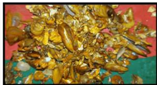
Figure 4 Dirt and shells in condenser
