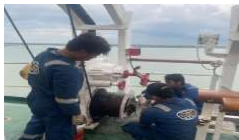
Figure 4. Crew deck work not using safety helmet
