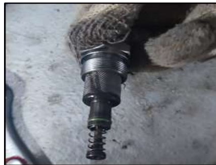
Figure 6. Cleaning strainer filter burner
