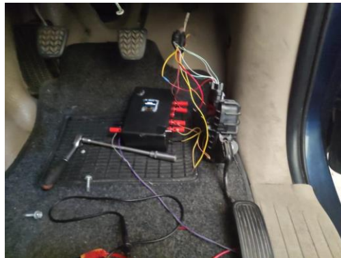
Figure 5. Installation of the Tool on the APP Sensor
