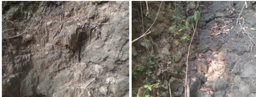
Figure 3. Joints formed in the landslide area
