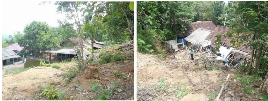
Figure 3. Karangtengah avalanche which resulted in the destruction of houses
