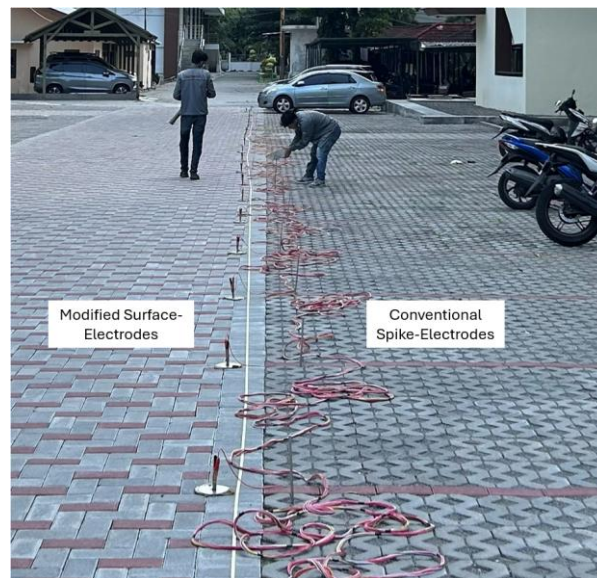
Figure 3. Test site conditions and electrode arrangement along the ERT survey line. The left side shows the application of MSE on the closed surface, and the right shows the application of conventional spike electrodes on the open surface
